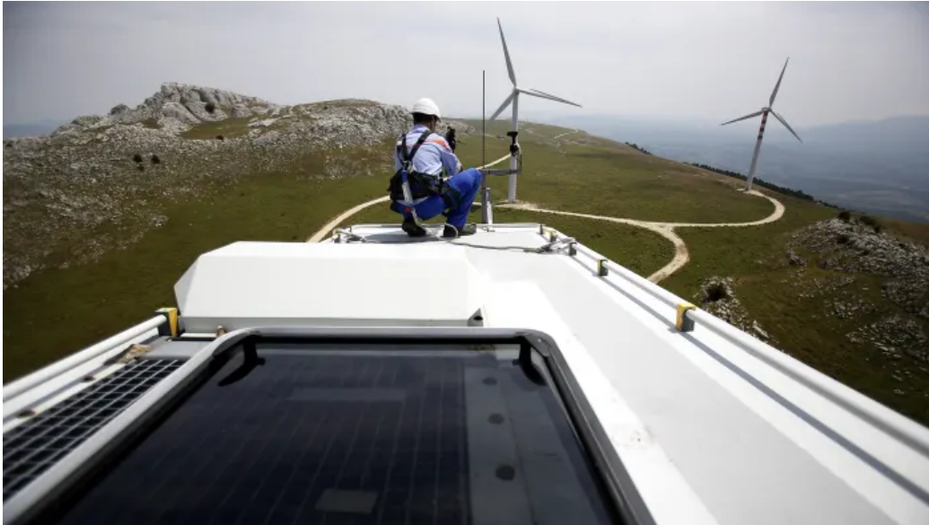
High tech: Maintenance work on a wind turbine in Italy © Bloomberg
