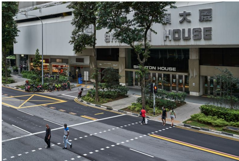
Shenton House on Shenton Way, an older part of the business district in need of rejuvenation.
